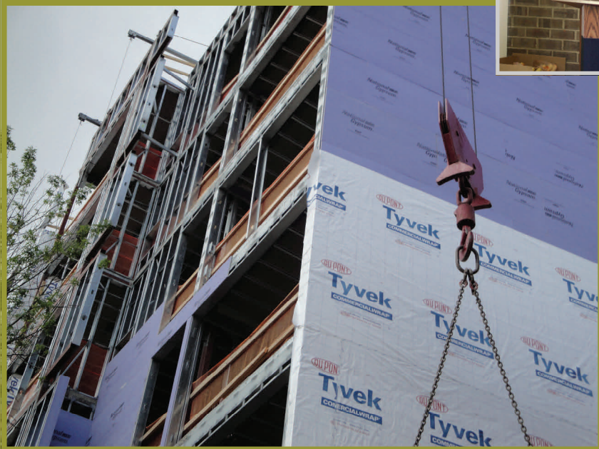
Photo Below: 3 Tree Flats Topping Off Ceremony
